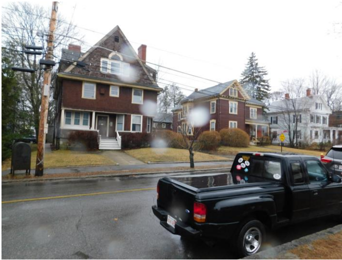
View from W. Emerson, Buildings 1 & 2
