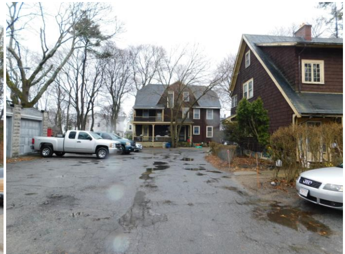
View toward building 4
