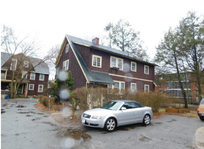
View toward building 3, building 4 in background
